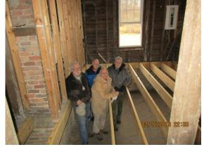
where the top of the joists were to stop. Paul had a laser level that we used in order set the band boards in place so that the floor in both the front and back sections of the house would be level with each other. Once all of these heights were marked, we used anchor bolts to fasten the band boards to the basic framing of the house.
